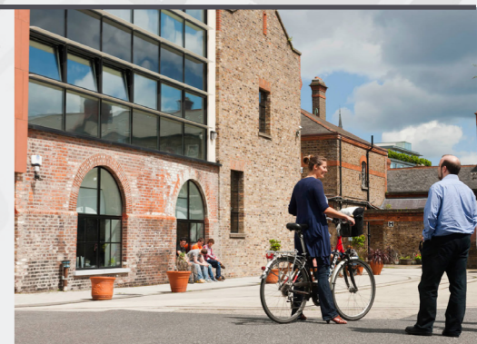
New Market Yard: A new City Square can replace the functionality of the Ladies' Market and include activation of the screened IW Pumphouse
