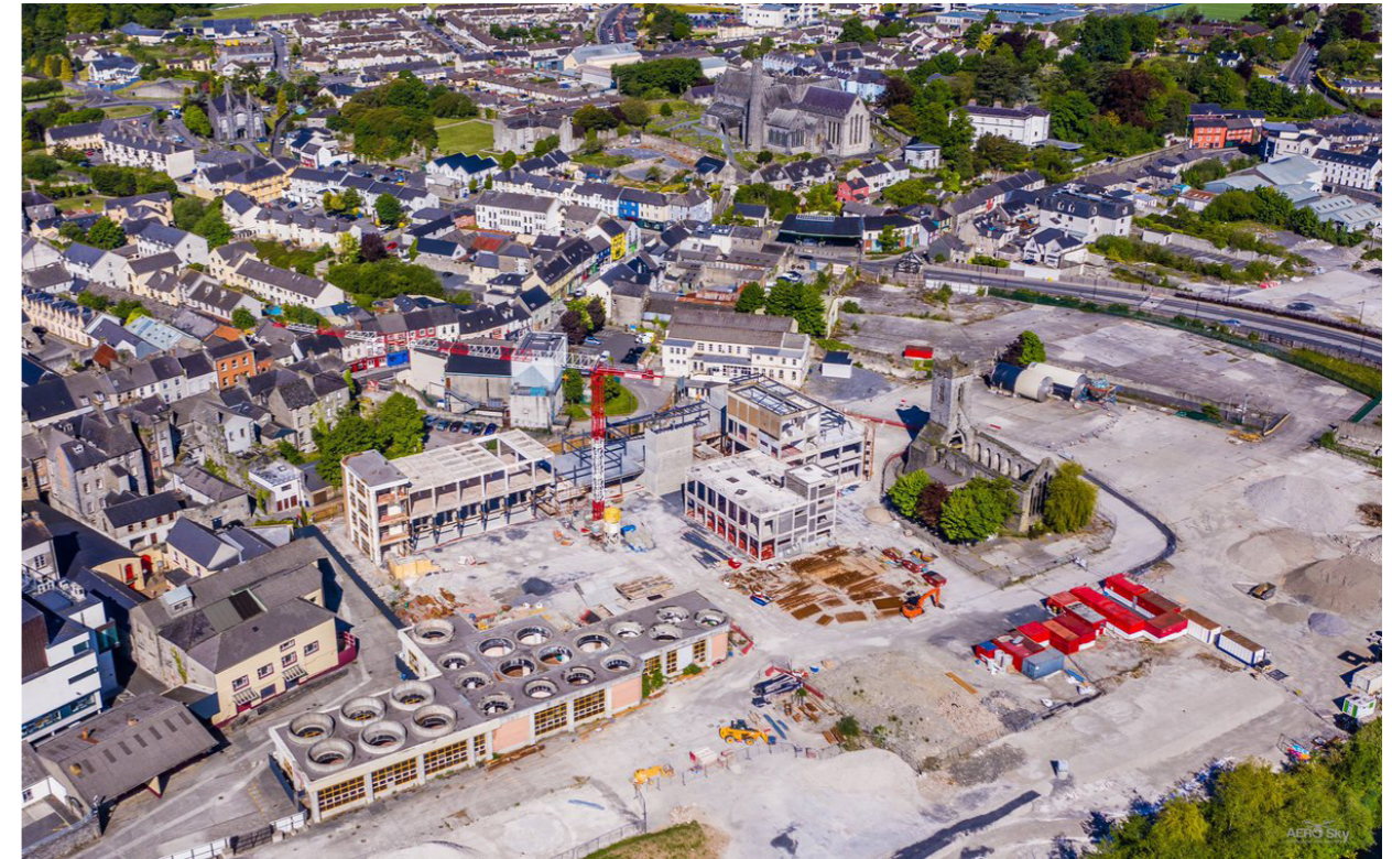
Aerial view of the former brewery before redevelopment began
